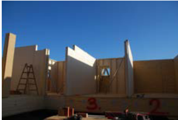
View of the erected interior walls already prefabricated on one side, the open compartments (picture on the right) will later be filled with hemp insulation mats and closed with 3-layer boards spruce.
