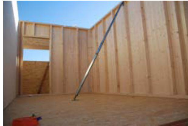
View of the erected interior walls already prefabricated on one side, the open compartments (picture on the right) will later be filled with hemp insulation mats and closed with 3-layer boards spruce.
