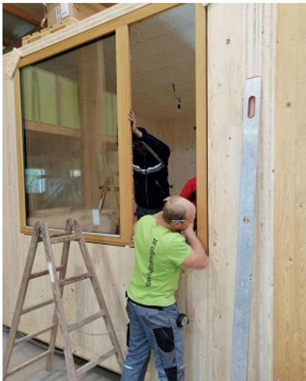
Interior joinery work from top left to bottom right: Assembly of the modular ceiling panels for the lower ceiling, installation of the frames for the interior doors, the installation of all windows and also the front doors are already done in the factory.
