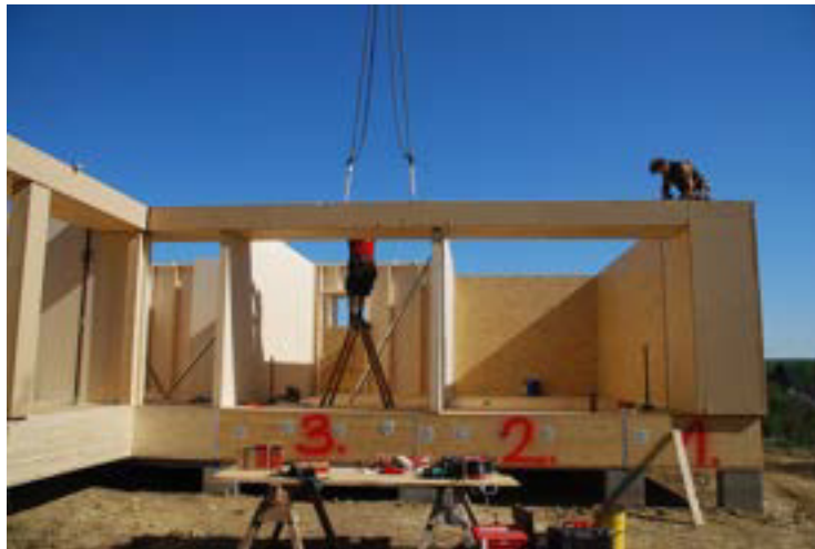
View of the erected interior walls already prefabricated on one side, the open compartments (picture on the right) will later be filled with hemp insulation mats and closed with 3-layer boards spruce.
