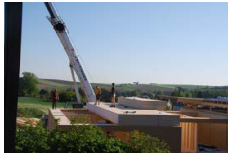
After the assembly of the overlays, the ceiling elements are moved and installed. Due to the prefabrication and the accuracy of fit of the individual elements, one residential unit (an atrium house) could be erected within one week including the roof structure.
